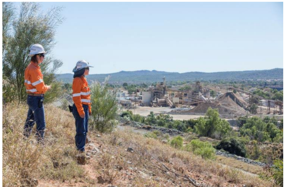
Figure 1 Overview of Processing Plant.
